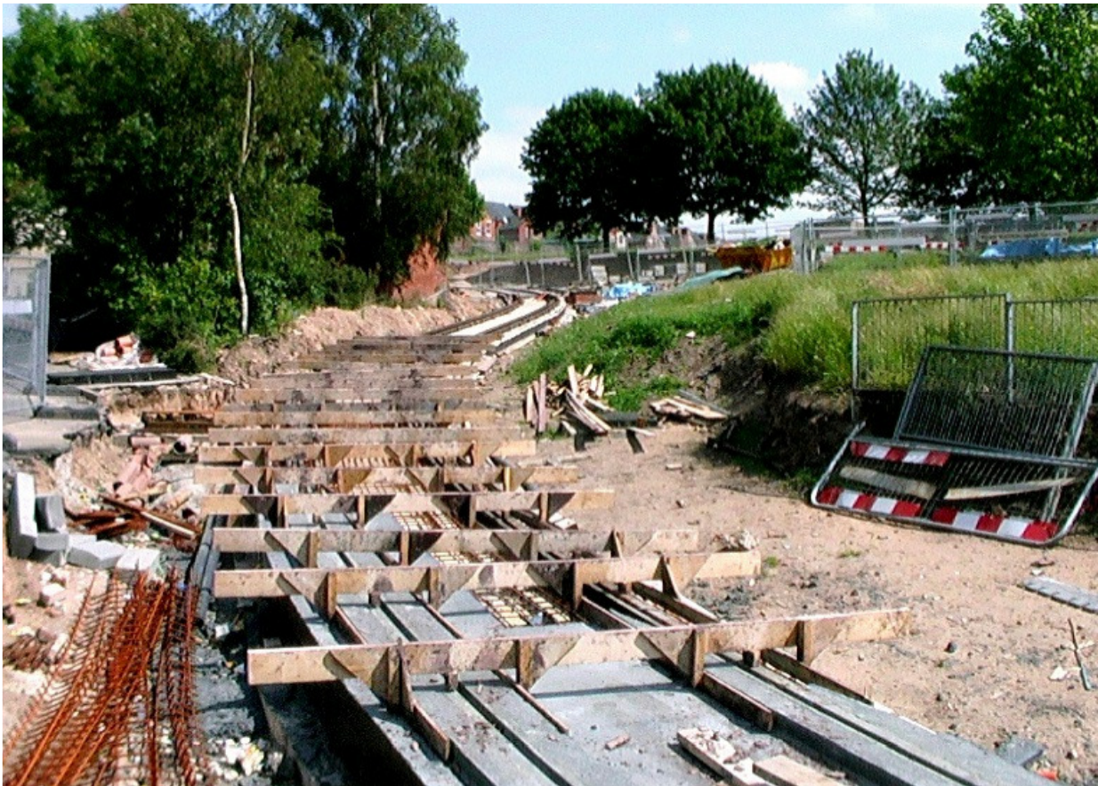
Figure 3.5: Concrete pour around the rails
