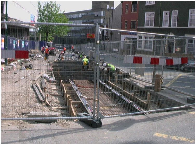
Figure 3.3: Reinforcement Mesh
