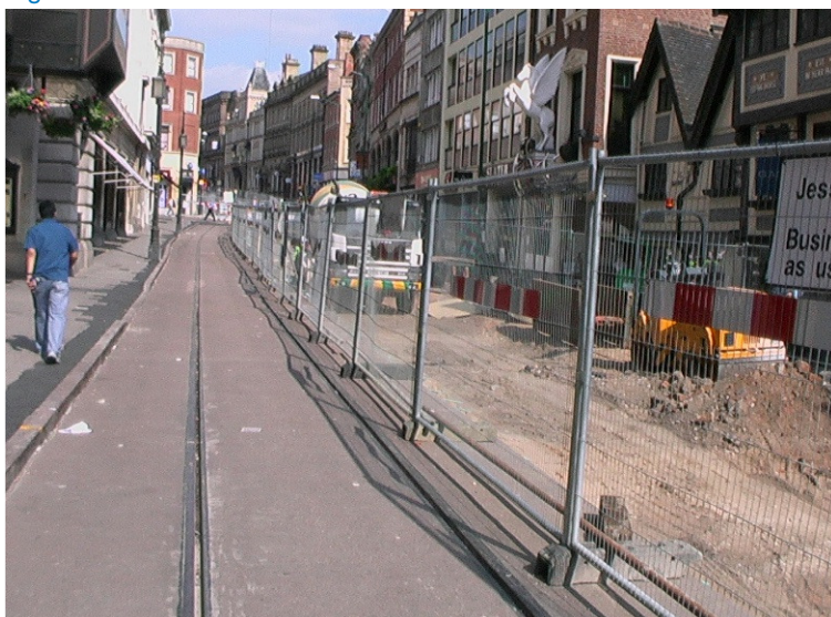
Figure 3.2: Sub-base material construction
