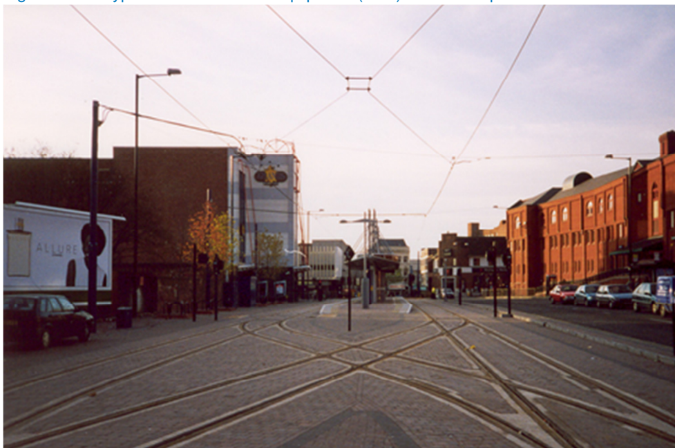
Figure 3.6: Typical Overhead Line Equipment (OLE) Wolverhampton Midland Metro
