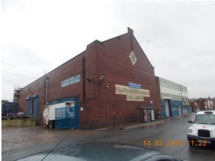
Photo 47: Industrial building on Fazeley Street
