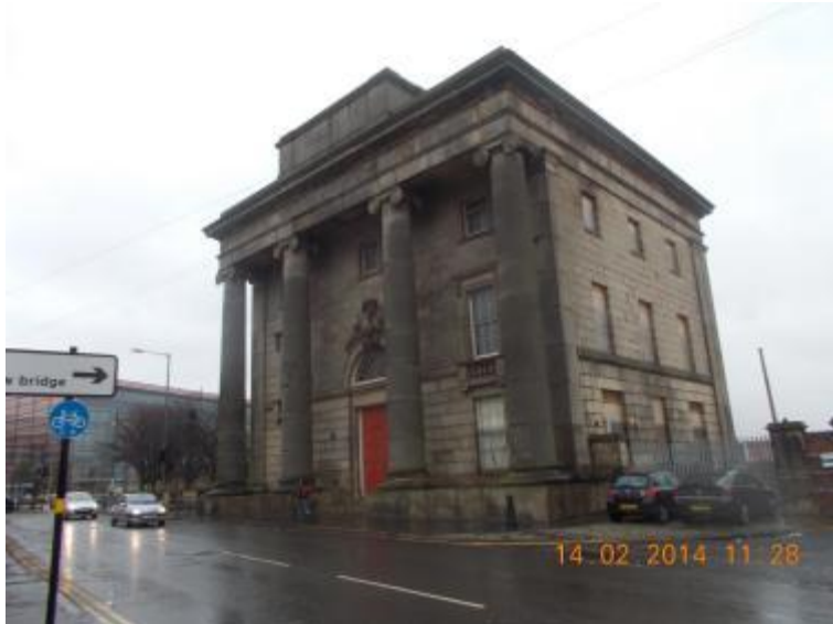
Photo 55: Former Curzon Street Station building
