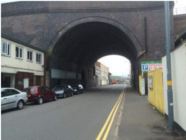
Photo 72: View north of Moor St railway line viaduct
