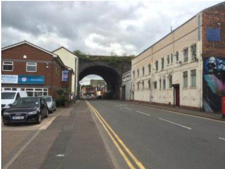
Photo 71: View south along New Canal Street, at Bordesley Street junction
