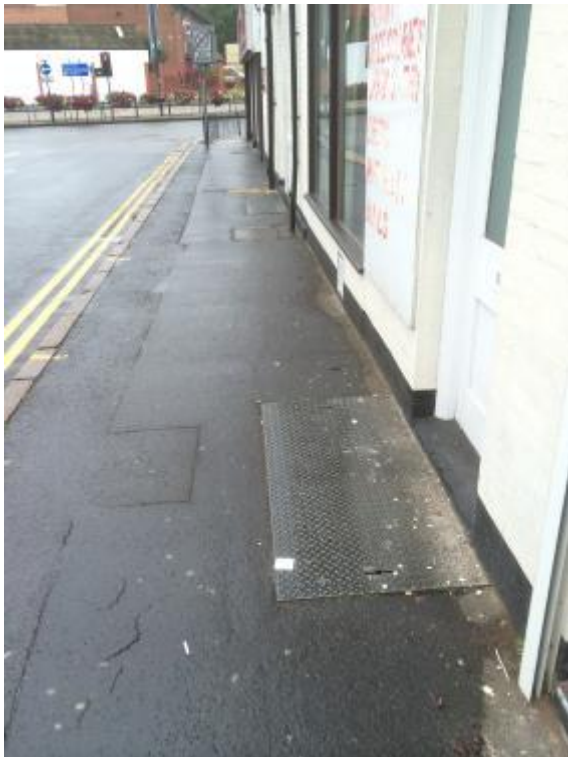
Photo 80: Suspected basements under existing footway (facing south)
