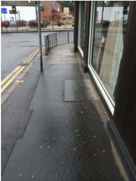
Photo 81: Suspected basements under existing footway (facing south)
