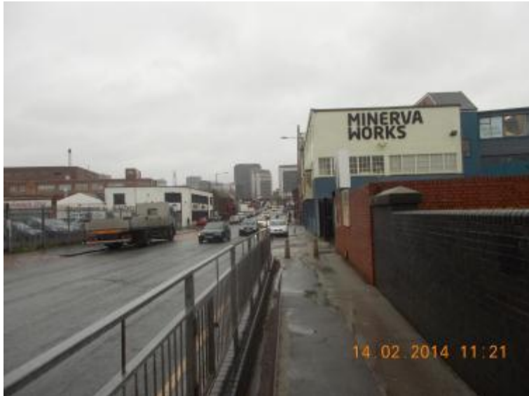
Photo 45: View west along Fazeley Street
