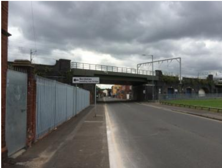
Photo 67: View south along New Canal Street towards New St railway line
